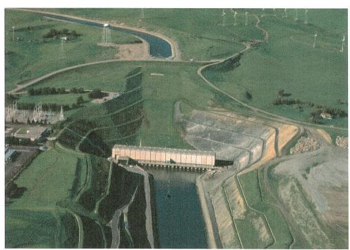
An aerial view of the Harvey O. Banks Delta Pumping Plant, the first major plant designed and constructed within the California State Water Project. The facility located in Alameda County has a number of pumps that lifts water into the California Aqueduct. (California Department of Water Resources)
